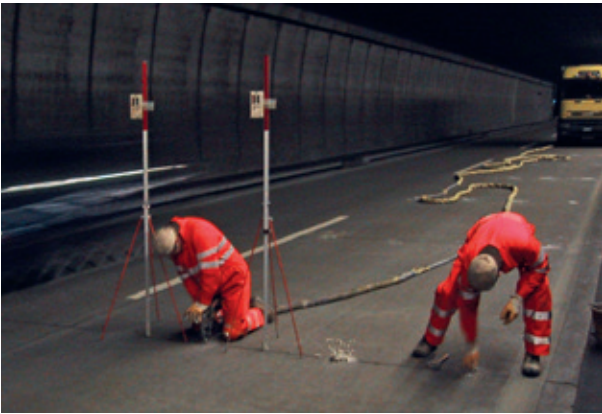
Tunnel Seelisberg A2
